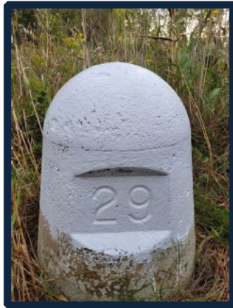
Typical frustrum shaped Reference Monument, MI/ON
